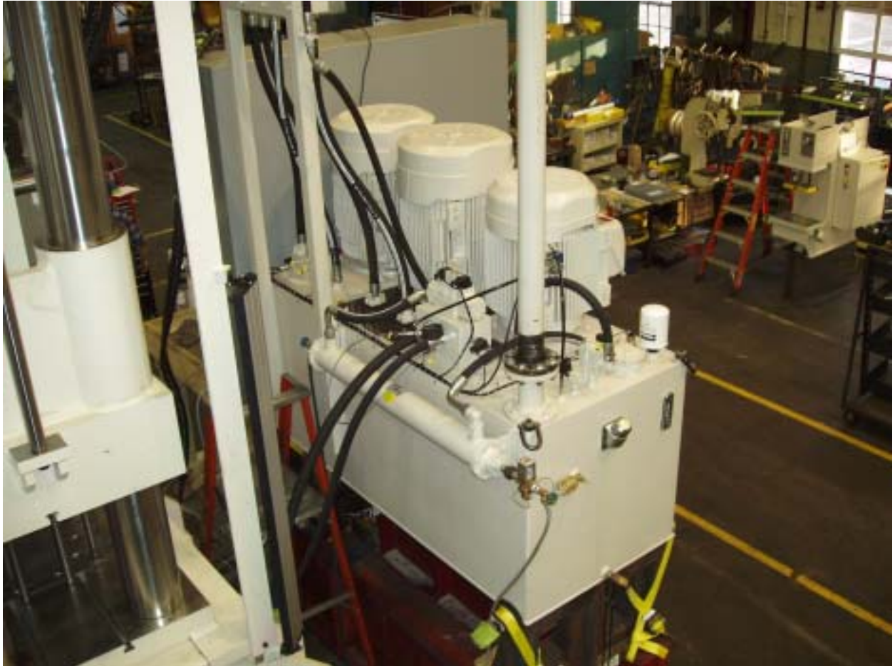
Overhead view of Main Power Unit.
